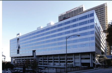
SUNTRUST PLAZA GARDEN OFFICES ATLANTA, GA 30303
