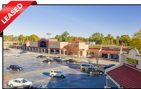
3720 BOILING SPRINGS ROAD
