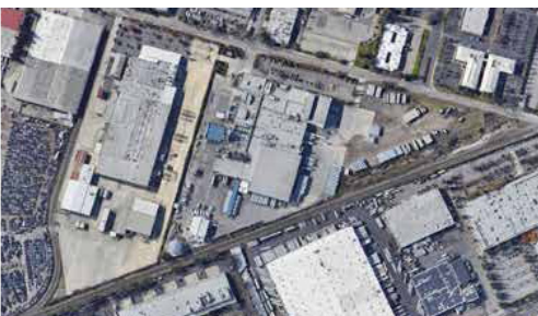
Hayward Logistics Center Two Class "A" Warehouse Buildings Estimated Delivery Q4 2021
