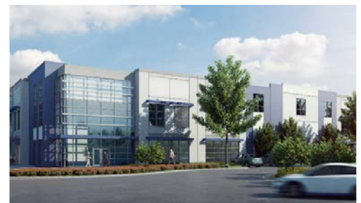
Class "A" Advanced Manufacturing Space 4 Buildings, 35% Pre-Leased
