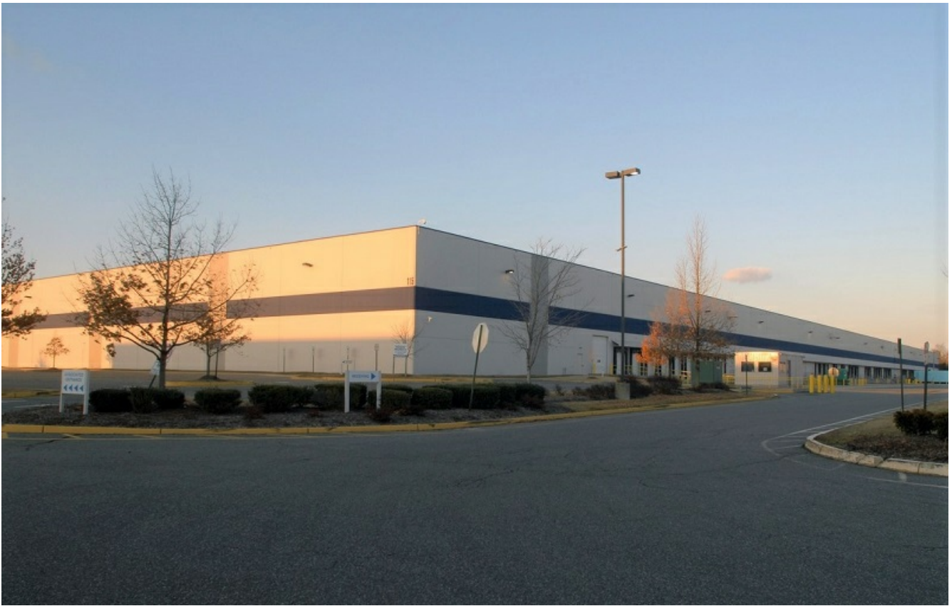
Lee & Associates' Dave Saltzman recently represented XPO Logistics in a 526,400-square-foot lease at 115 Interstate Blvd. in South Brunswick. — Courtesy: Lee & Associate
